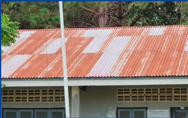
▶ 補修前の校舎屋根
